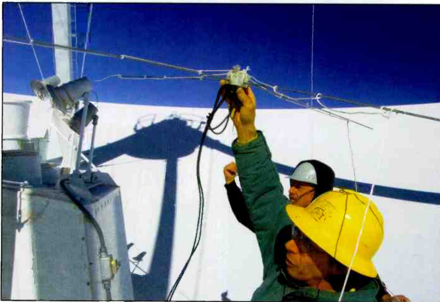
Photo J. A closer view of the 74-MHz dipoles also shows the balun box. The team is about ready to raise the dipole with the ropes.
