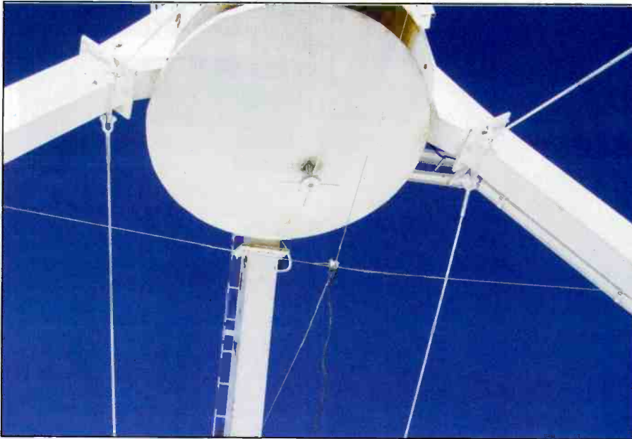
Photo I. Ropes hold up the 74-MHz (4-band) antennas. "These are good old-fashioned dipoles, also arranged to provide the two orthogonal polarizations and in the same orientation as the P-band," writes NA5N.
