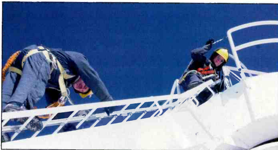
Photo M. In hot weather, heat issues are multiplied exponentially when the team is wearing the required overalls and fall-arrest safety harnesses to climb to the apex.
